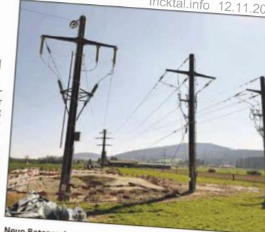
Neue Betonendmasten in Rheinfelden. Foto: fricktal.info 12.11.2025
